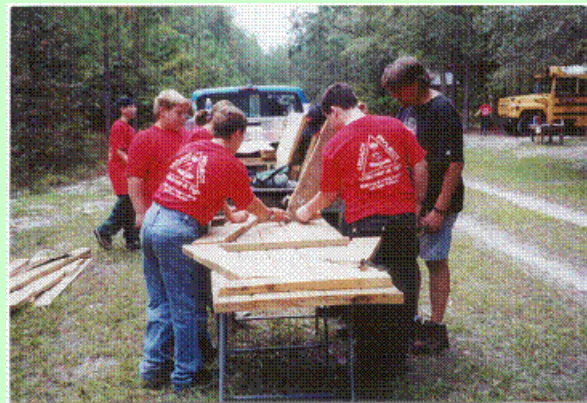
Water Action Volunteers: students building picnic tables at J. P. Hall Nature Preserve.
